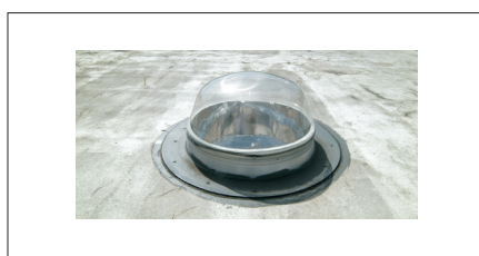
Figure 4 Flat roof flashing installation
