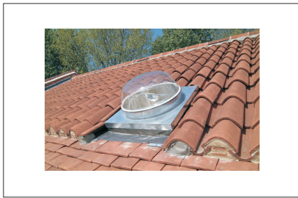
Figure 5 Curb mount installation
